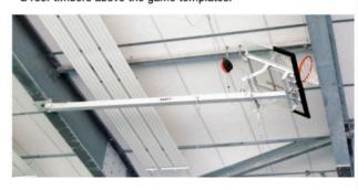
IMPORTANT: This solution is not always possible. Roof timbers must be placed out enough and thick enough in order to place board and ring in between. Strengtheners must be useful because of the space in between roof timbers.
